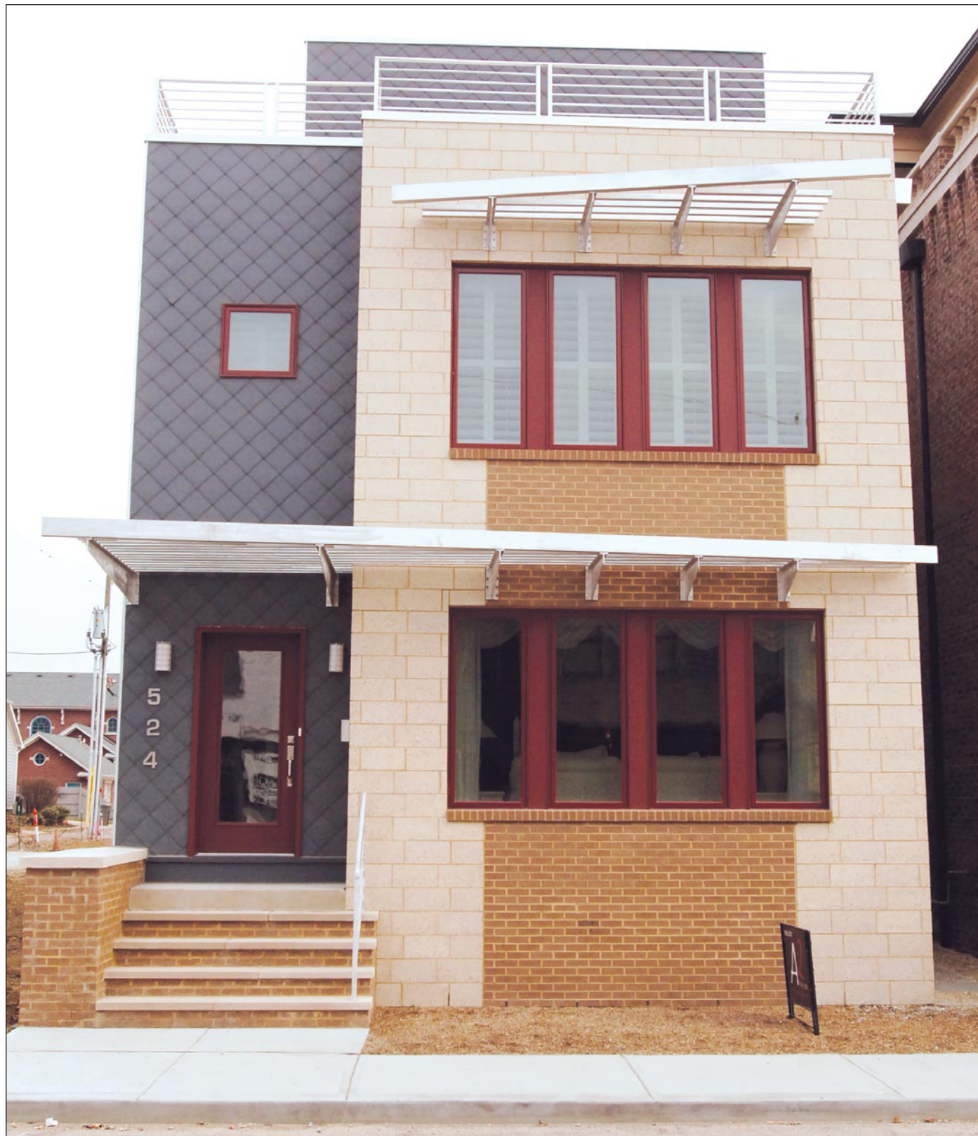
The Reiter home's exterior features a blend of concrete block, brick, slate-like fiberglass squares and stainless steel accents.
